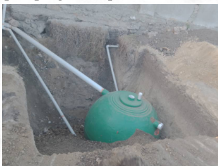
Septic tank installed at SiCC
